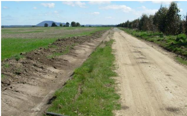
*This photo was taken on Sunday 25<sup>th</sup> September. Only a couple of weeks ago the track was under water. The drainage channel, the crushed rock and the recent dry weather has saved our scalps!!!*
