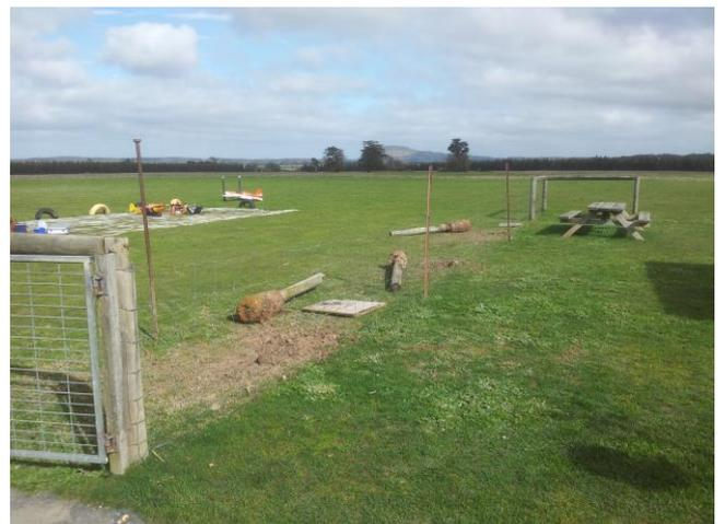
*Treated pine posts removed. Note the concrete which necessitated digging them out – at least the ground is soft.*
