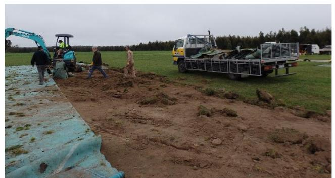
The Kobelco with Martin at the controls made light work of a rather daunting task. When the matting was laid the grader went along the edge of the strip with the blade on an angle to dig a trench. The edge of the matting was laid in the trench then the grader back filled locking it into place. After several years of grass growing through it, it was just impossible to pull out by hand.
