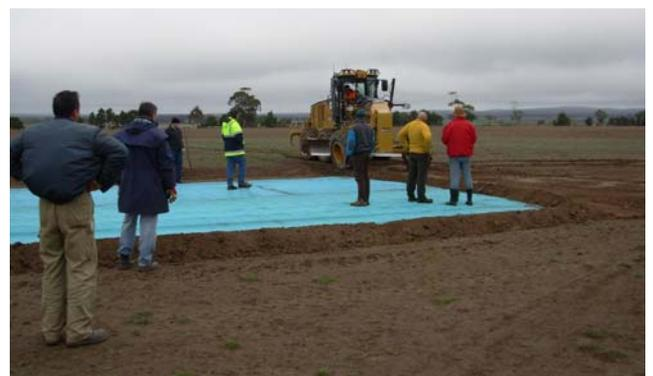
*It's about 10:30AM, field has been graded and matting laid out ready for the edges to be buried. Craig is backfilling the western end with the grader blade under the scrutiny of many watchful eyes.*
