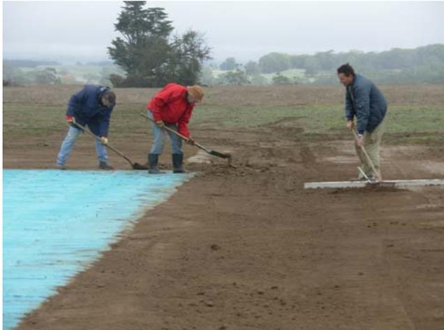
Once the backfilling was done by the grader it was a matter of smoothing the edges. Noel had his straight edge clamped to his rake which worked well.
