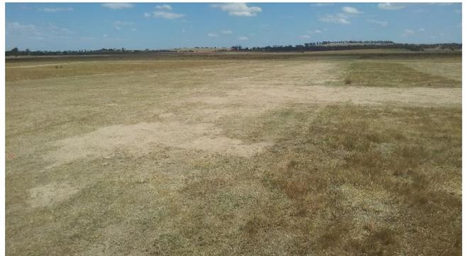
*The main N/S runway with top soil filling holes & depressions mainly along the western side. Some soaking rain would be nice now to consolidate the fill.*
