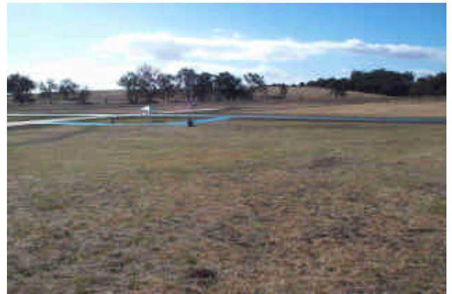
The runways at the Twin Cities Club new field. The surface was a high density woven plastic mat obtained from the nearby paper mill.
