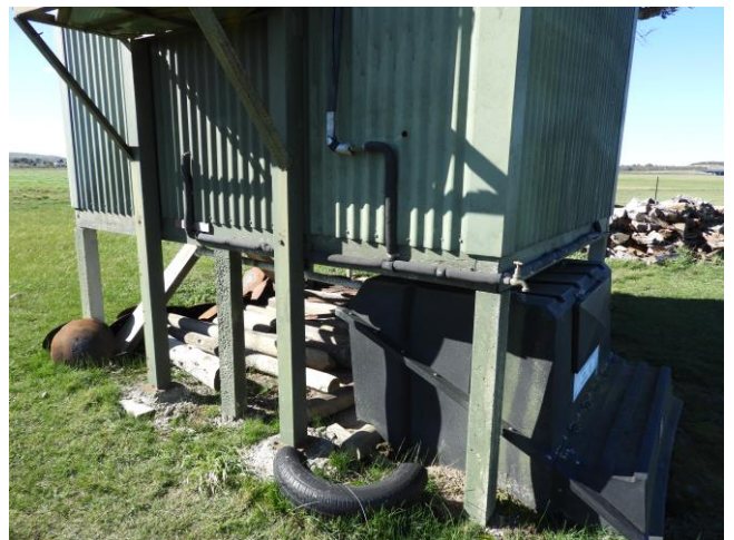
Max fitted new copper pipe along base of toilet.
