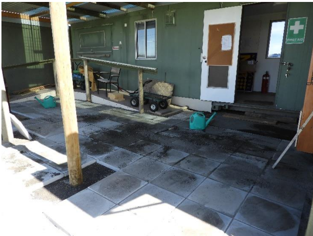
Most of the slabs had been laid by midday with the few that required cutting in remaining for the following Sunday. (Wednesday 4 th October.)
