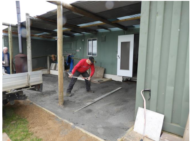
The all-important preparatory work getting the area flat ready for the slabs to be laid. (Sunday 1 st October).
