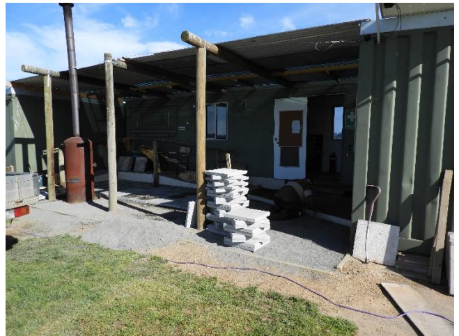
The slabs from the first trip on Tuesday 3 rd October. The pallet of 60 weighed just on 1 tonne. (Wed 4 th October).
