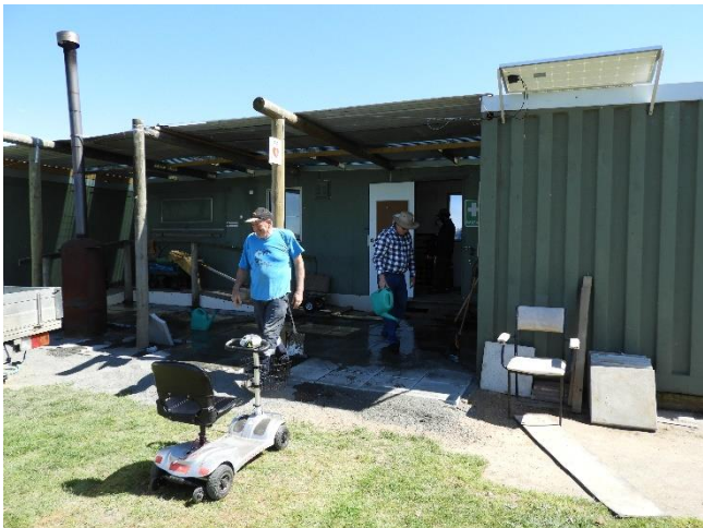
Secretary Nigel was sweeping the blue metal dust in between the slabs and wetting it in to help bed them down.
