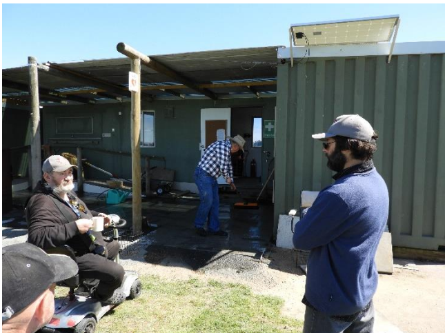
Paul and Ricky also popped in on the day to lend a hand. The mounting bracket for the Defibrillator machine was fitted inside as well as the outside sign on the post. (Wednesday 4 th October.)
