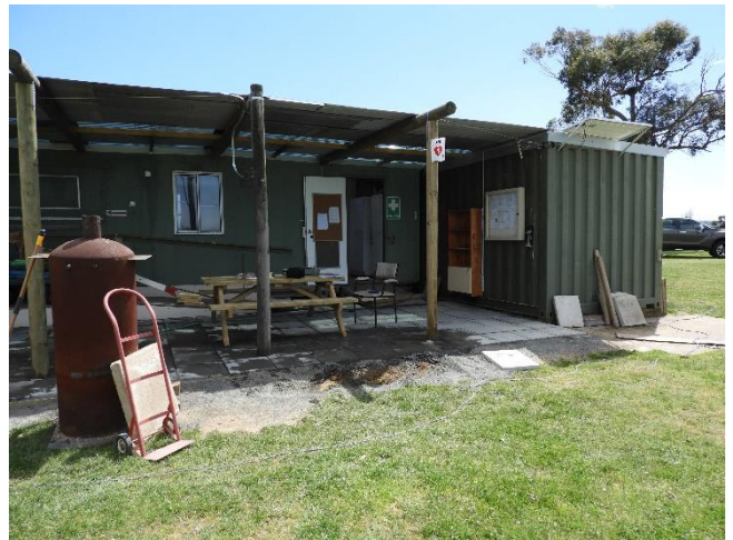
Murri finished off laying the pavers that needed cutting in on Sunday 8 th October and then finalized the job the following weekend. (Photo taken 8 th October.)
