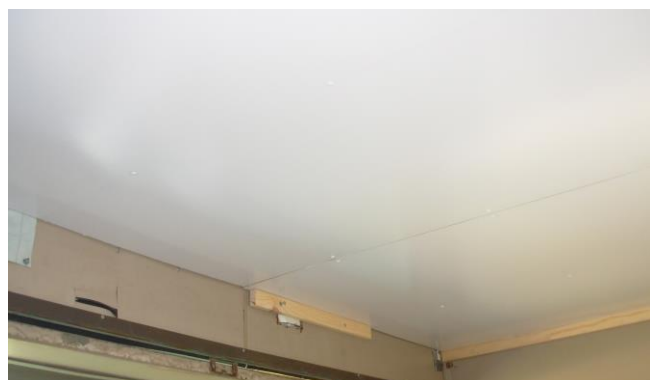
The new lining has been glued & screwed to the ceiling in the servery area. There will be a 2x1 timber cornice all the way around and the holes in the wall will be covered prior to painting.
