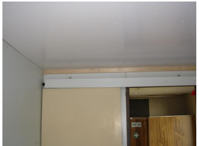
The new ceiling lining makes a huge difference already. The walls which are steel clad inside will be painted as well after several holes which were cut for various reasons over the years are covered.
