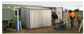
By days end we had the structure in place. On Monday Max & I (Roger) went out and finished it off with flashing and spouting. The following Saturday the 18<sup>th</sup> a couple of vents were fitted to the roof, it was also cleaned and painted making it look quite respectable. Just needs a louvre window to finish it off.
