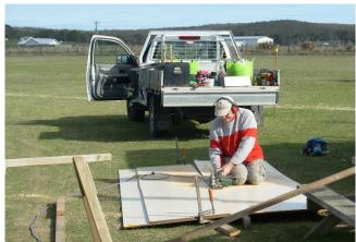
Murri cutting the Laminex high density compressed board for the servery ramp. The material is extremely tough and makes a saw work really hard. Ideally a diamond tipped blade is should be used.
