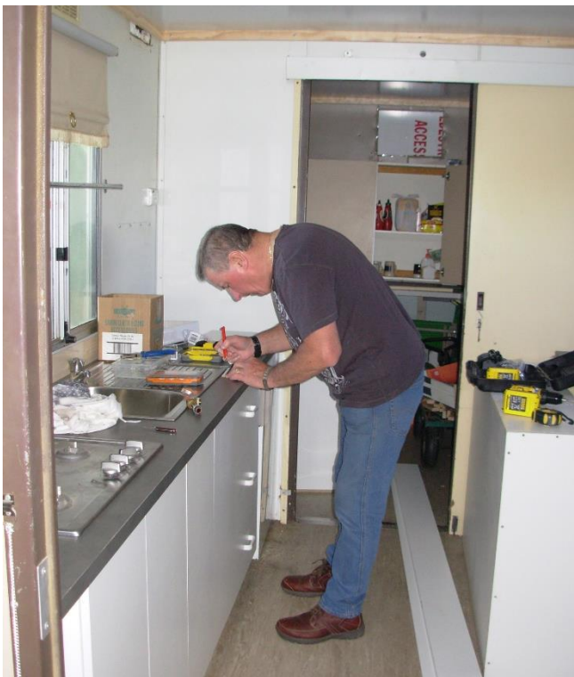
Graeme assembled the cupboards and prepared the benchtops at home. The benchtops involved gluing & trimming the Laminex then cutting out the holes to suit the sink and stove.
