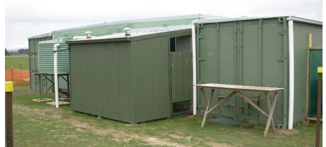
The BBQ enclosure (aka the chook shed) erected on Saturday 11 th July was finished off the following Saturday (18 th ) including a paint job to make it blend in.
