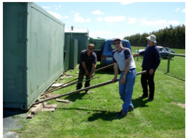
Some tossers trying to lift a 10 tonne container with a crow bar and a couple of lengths of pipe.
