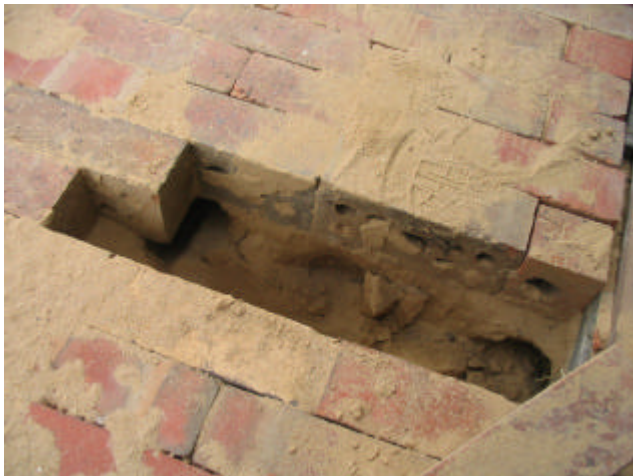
The damage done by a four legged rodent.
