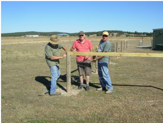
Peter E. is tying off the strainer wires with assistance (or maybe hindrance) from Glenn & Wayne.
