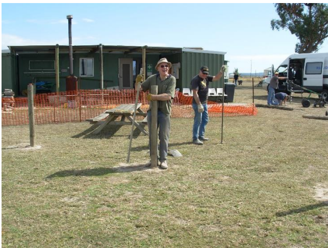
Secretary Jeff is stomping in the backfill around the posts. El Presidente Graeme is holding up the stomper.
