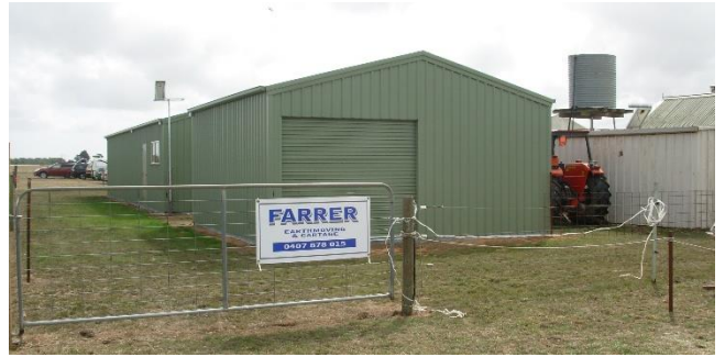
The two new sheds at the Warrnambool field with the smaller machinery shed in the foreground. The old structures to the right are to be dismantled at some stage.
