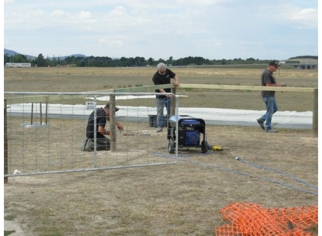
Max & Peter E. are attaching the diagonal strainer wires tying them off with a gripple.
