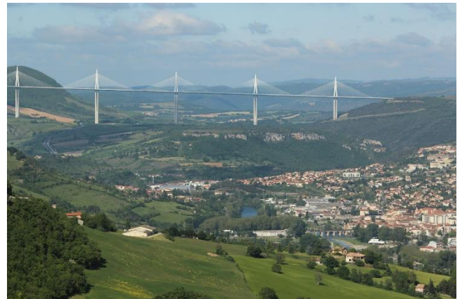
The Millau Viaduct (French: le Viaduc de Millau), is a cable-stayed bridge that spans the valley of the River Tarn near Millau in southern France. Designed by the French structural engineer Michel Virlogeux and British architect Norman Foster, it is the tallest bridge in the world with one mast's summit at 343.0 meters above the base of the structure. It is the 17 th highest bridge deck in the world, being 270 metres between the road deck and the ground below. The Millau Viaduct is part of the A75-A71 auto route axis from Paris to Béziers and Montpellier. The cost of construction was approximately €400 million. It was formally inaugurated on 14 December 2004, and opened to traffic on 16 December. The bridge has been consistently ranked as one of the great engineering achievements of all time. The bridge received the 2006 International Association for Bridge and Structural Engineering Outstanding Structure Award. (Information sourced from https://en.wikipedia.org/wiki/Millau_Viaduct )
