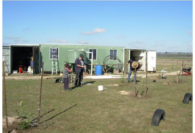
R to L. Peter Evans, Graham Waterhouse & Cato Werner tying the pittosporums to the fabricated wire sheep barriers. Yes there are sheep in the paddock but nothing like the numbers we had to contend with at Yendon.
