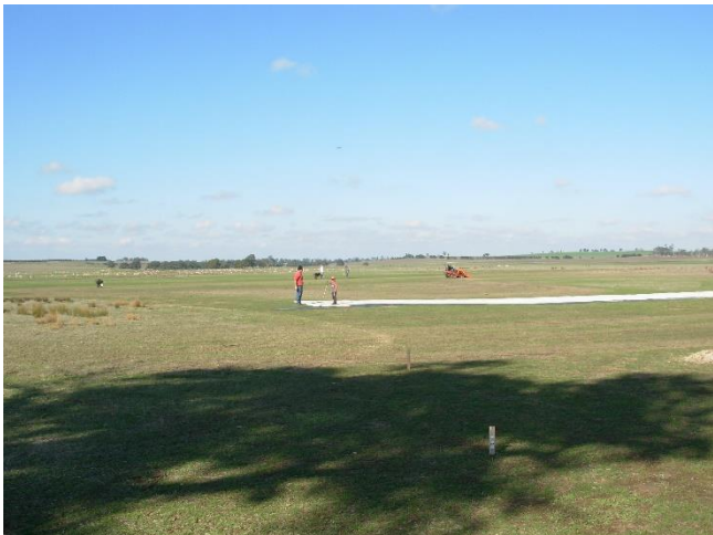
Graeme on his Kubota tractor spreading top soil on the runway low spots. Members also raking by hand to fill small holes. This time the top dressing was more selective and used bought soil rather than just spreading the fill that was available to us in the paddock like we did last time.
