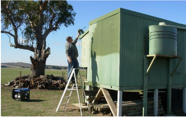
Mat spraying the walls of the toilet.
