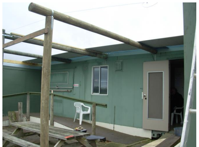
Murri has been working on the roof between the containers and kitchen. So far there's a half width strip of laser light and full width of iron on at the moment. There will be a full width strip of laser light going on next to augment the half width strip of laser light adjoining the kitchen followed by the rest of the iron. Paul Ruddle had some old iron at home that he kindly donated to the club.
