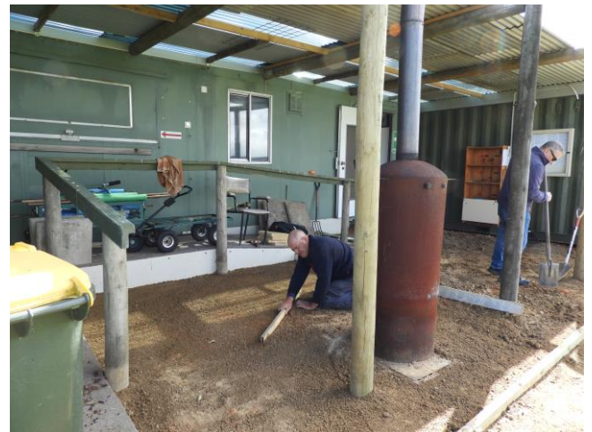
Murri is levelling the gravel which had been roughly laid a few weeks ago. It had compacted quite hard around the heater and took a bit of breaking the surface so it could be levelled.
