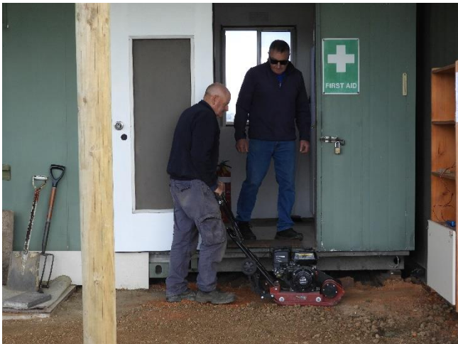
Nigel's mate had a whacker that we were able to borrow to compact the gravel. Some might suggest there are three whackers in this photo but the editor doesn't think that.
