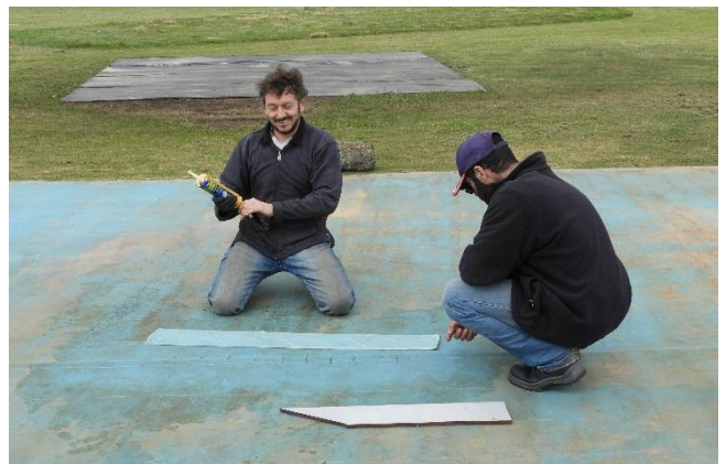
Looks like the job's done – fortunately the adhesive gave a reasonable bonding after about 10 minutes and assisted by moister.
