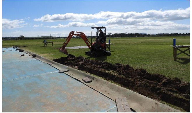
Tom digging the trench along the eastern boundary.
