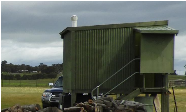
And the turbo vent all back in place doing what it does best.
