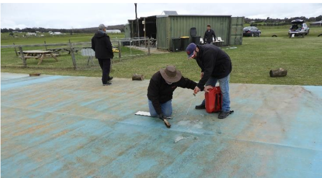
There was a frayed section so a patch was glued on top. Peter E. and Ricky cleaning ready for sticking on patch.
