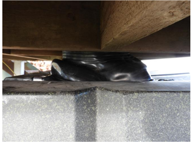
The new Dektite seal in place.
